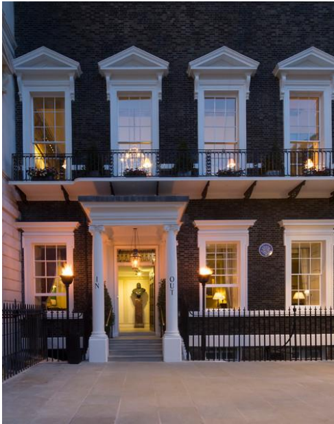
St James's Square Entrance
