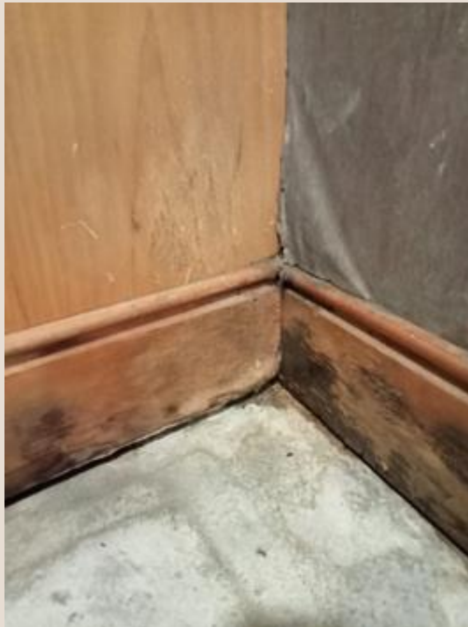
Leaks from walls at bowling area
