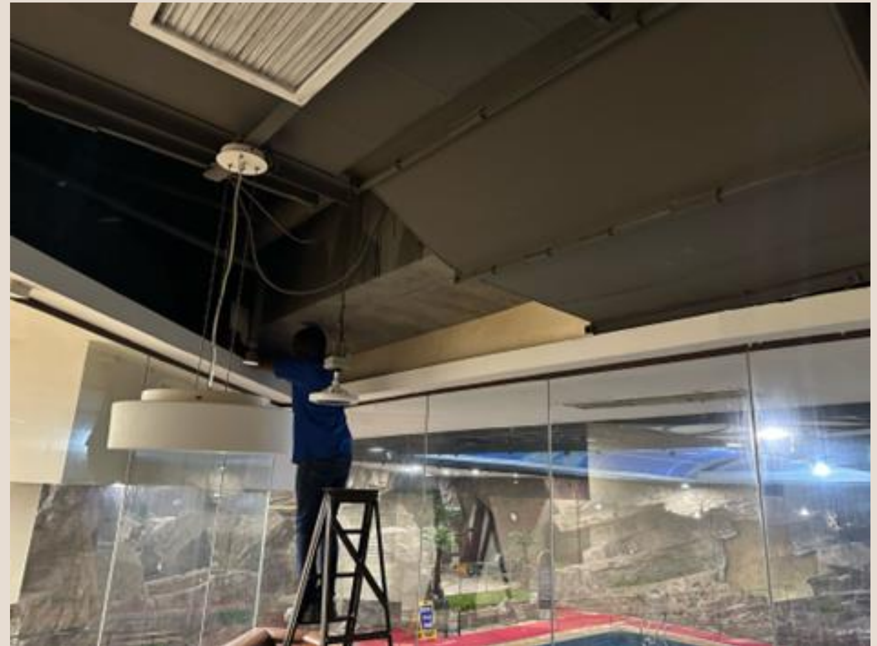
Sealing up the ceiling gaps along spaces to improve air quality
