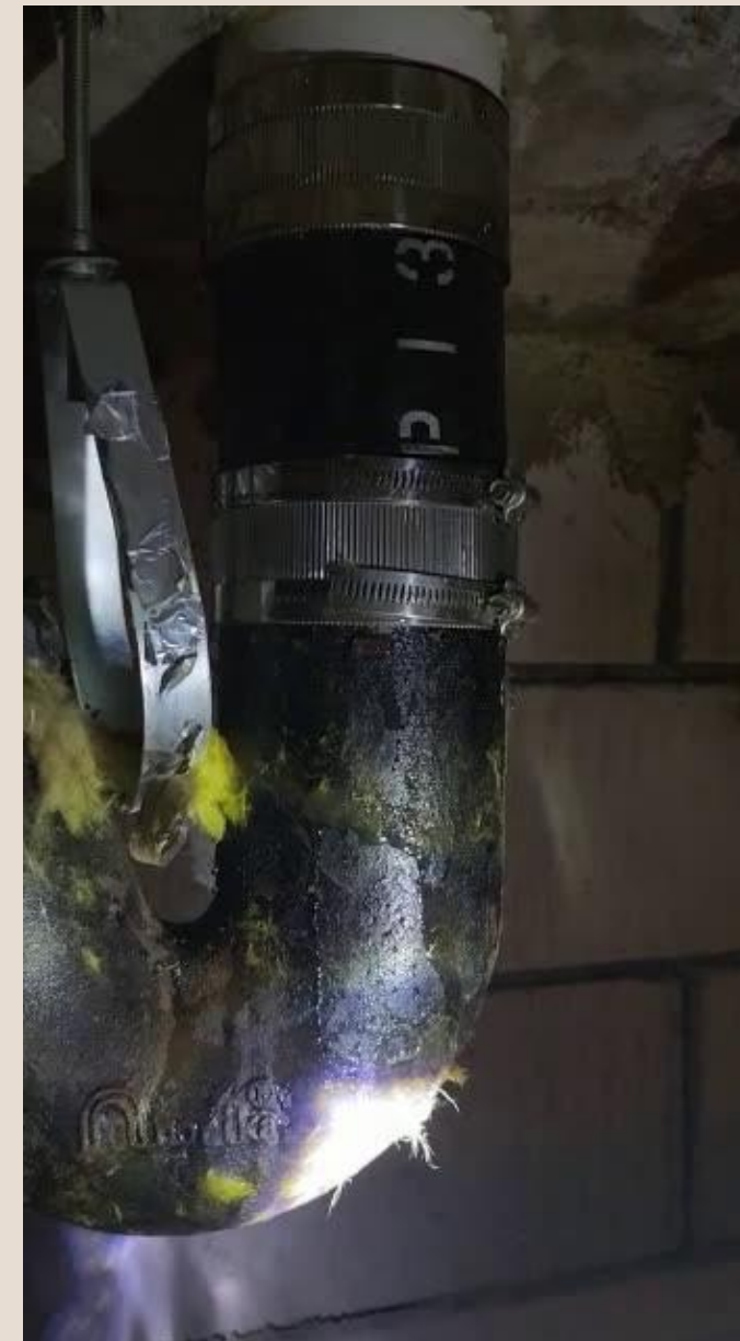
Leakages caused by Waste pipe corrosion (high occurrence)
