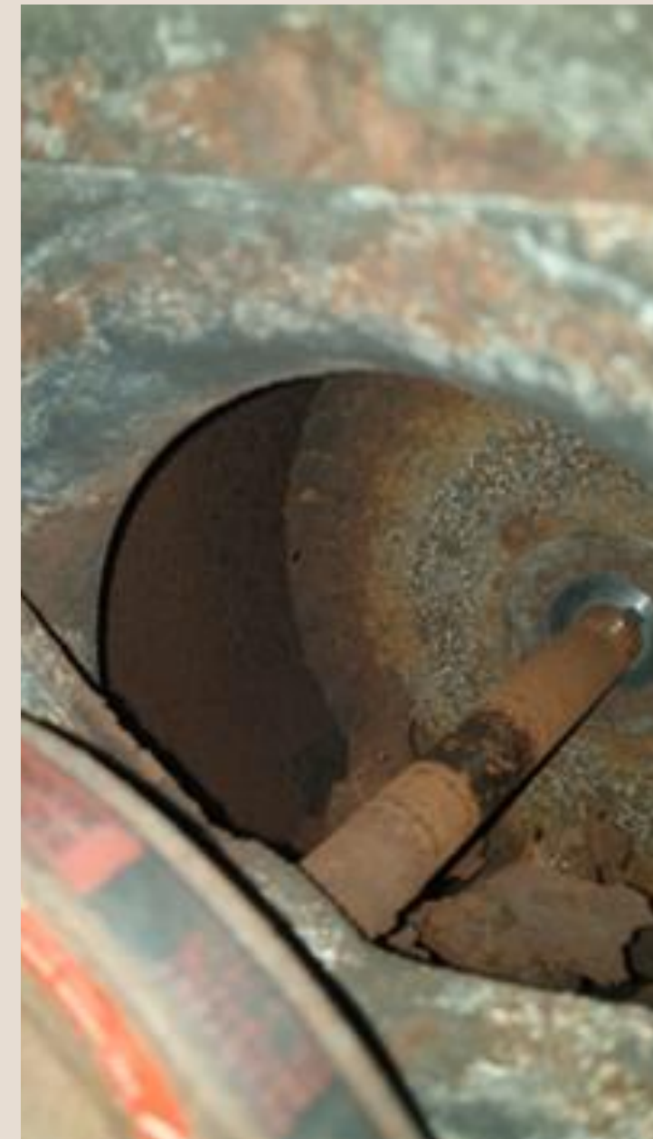
Air-con air handling unit (AHU) badly corroded
