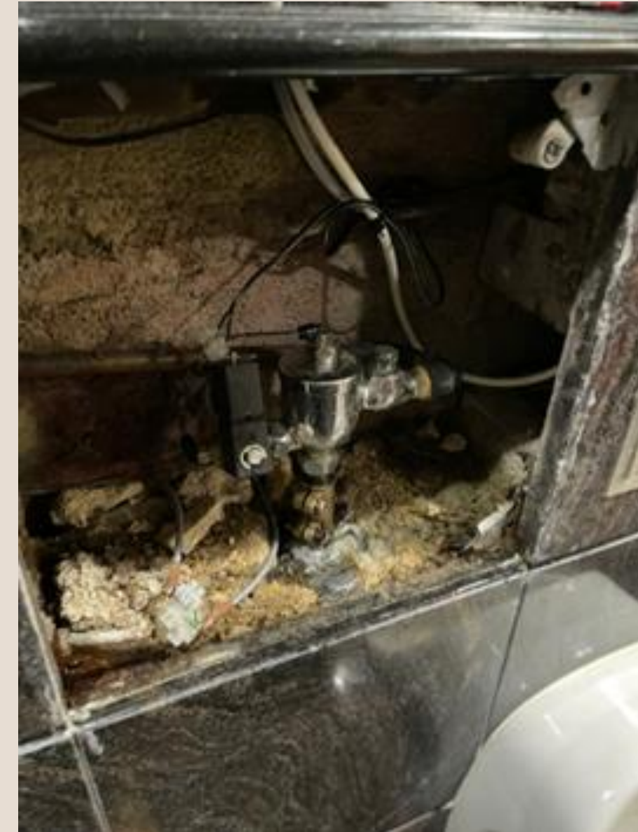
Faulty flush sensor (high occurrence)
