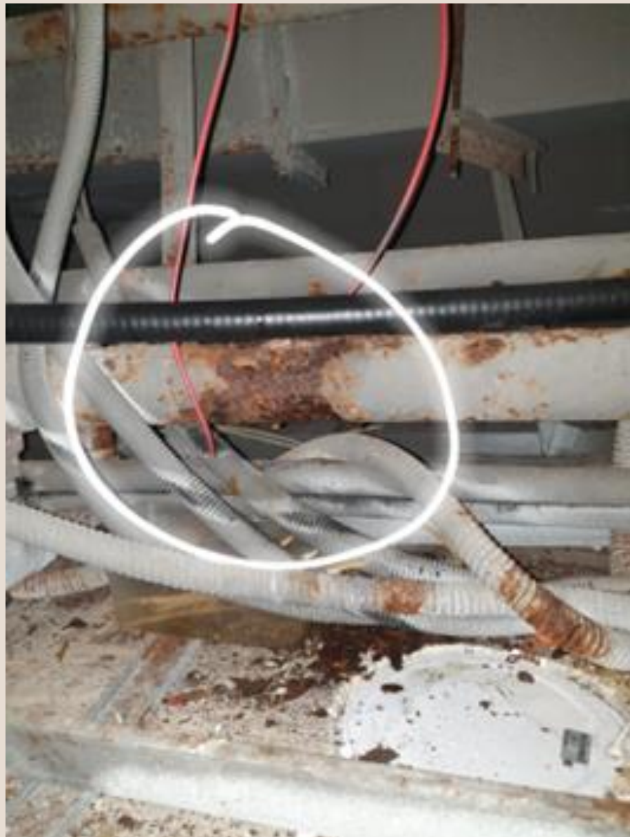
Sprinkler pipe burst at B1 Poolside Cafe due to heavy corrosion
