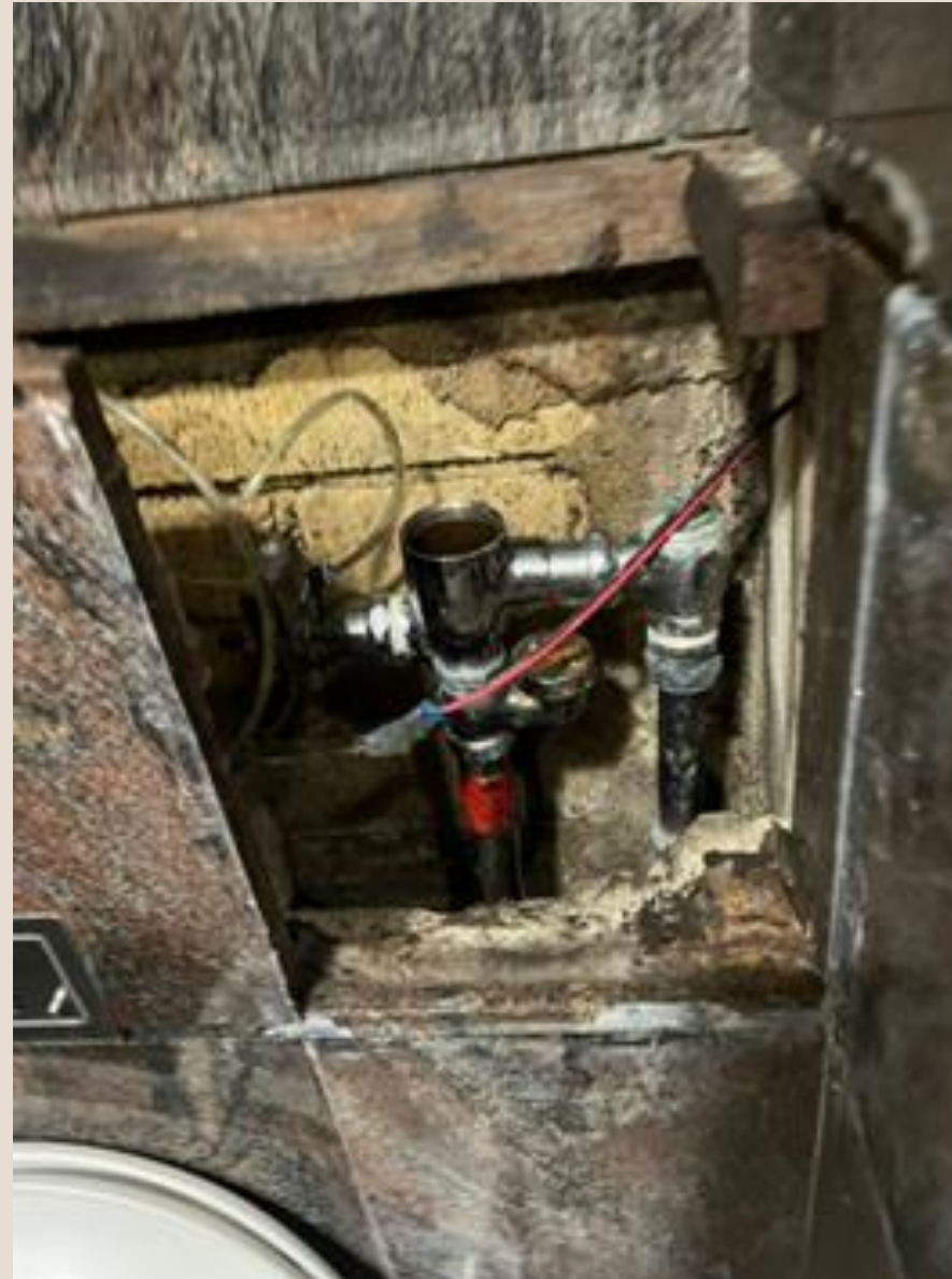
Faulty flush sensor (high occurrence)
