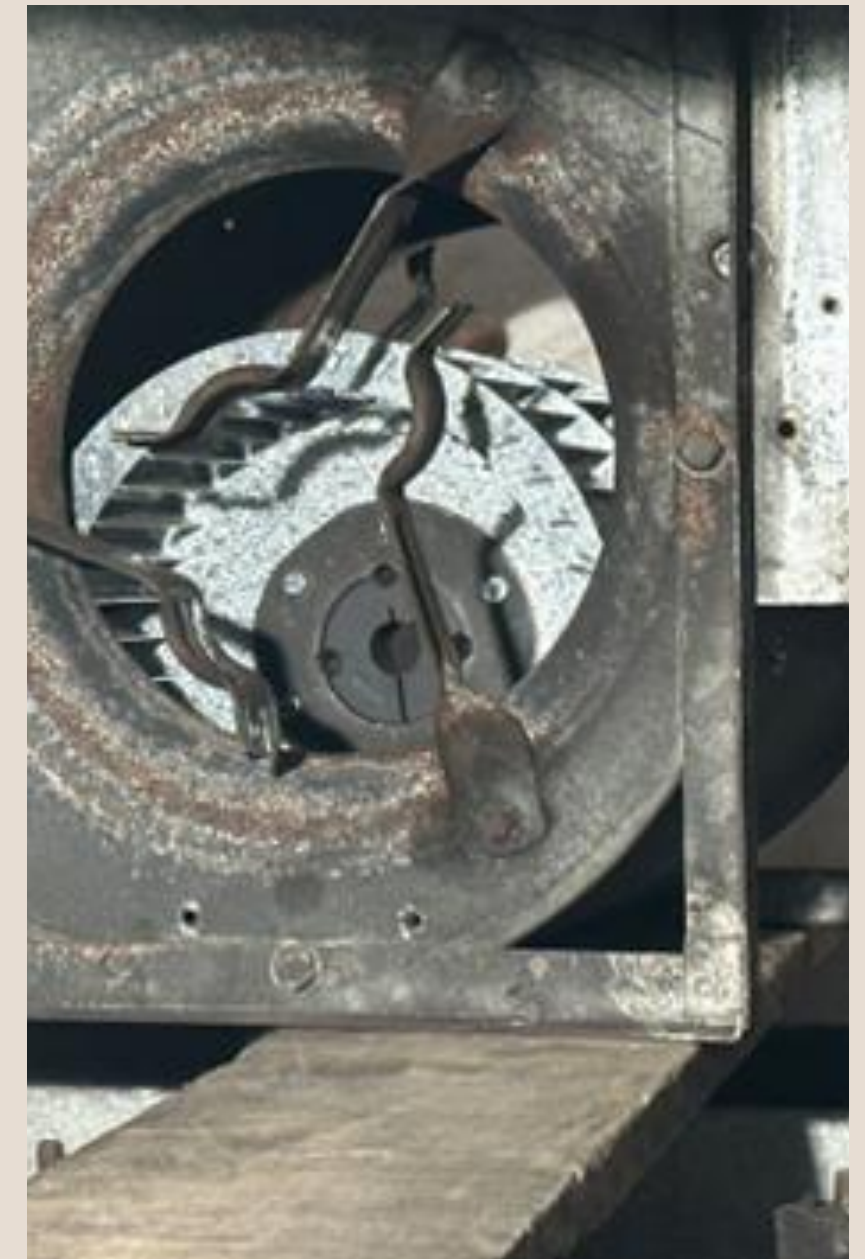
Air-con air handling unit (AHU) badly corroded
