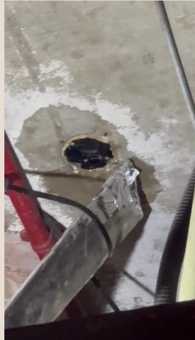
Leaking from level 3 to level 2 corridor (high occurrence)
