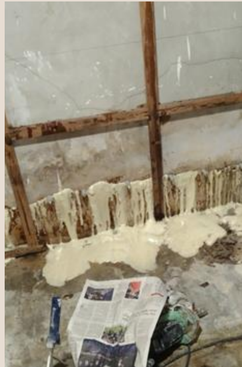
Leaks from walls at bowling area
