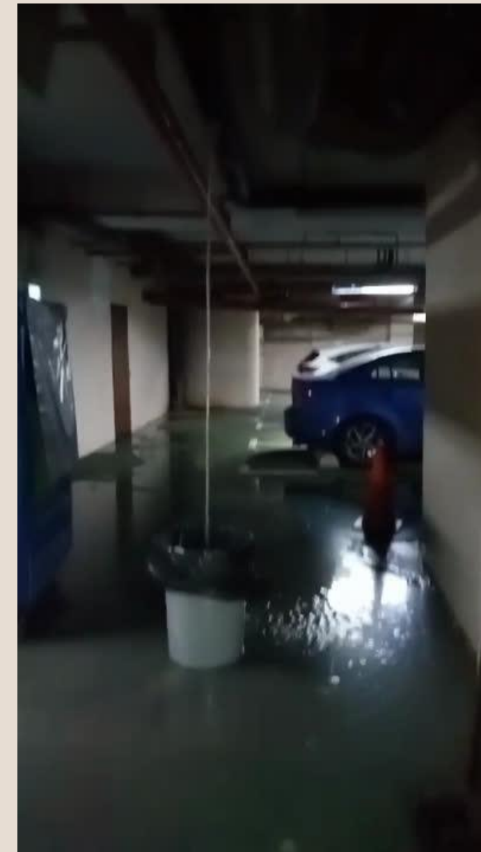
Leakages caused by Waste pipe chokages (high occurrence)
