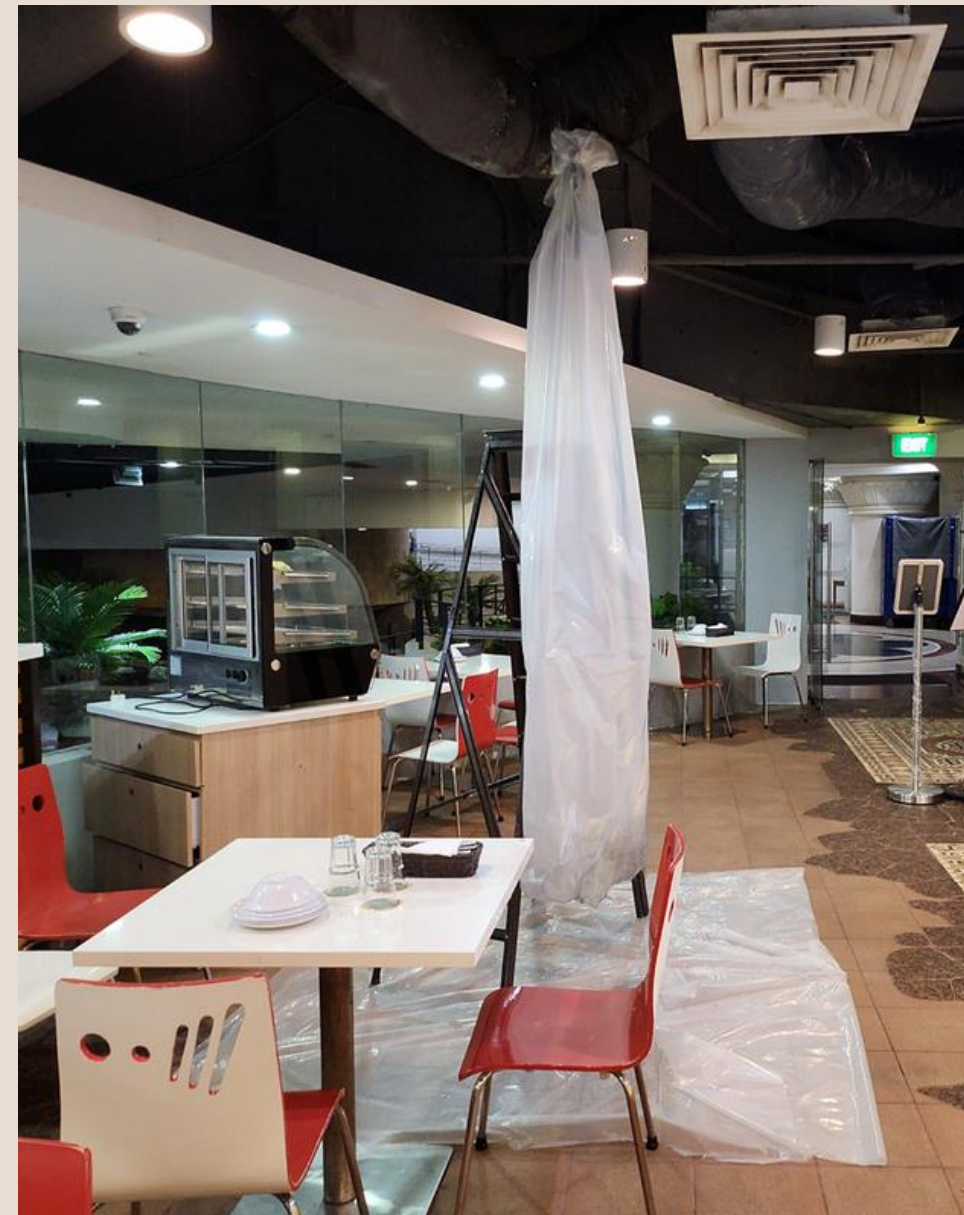
Sprinkler pipe burst at B1 Poolside Cafe due to heavy corrosion
